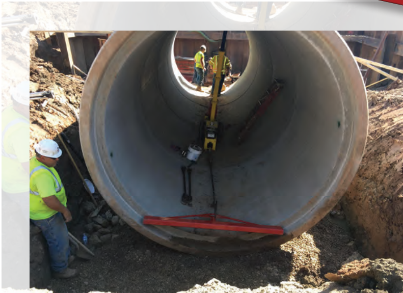
The optional RCP Long Cross Bar positioned in the culvert.
